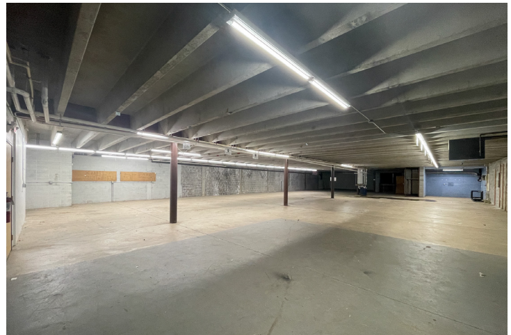
Basement ceiling measures 8'11" at lowest point.
