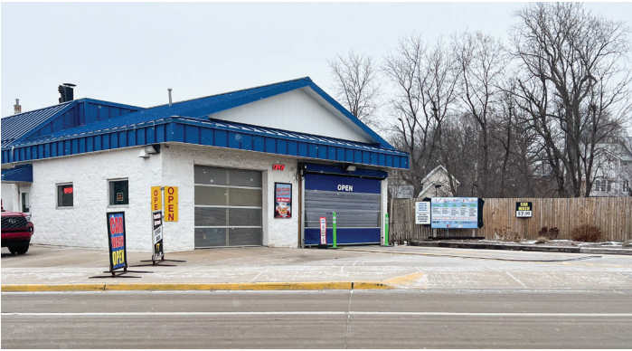
Car wash entrance on Hartwell (faces south) Detailing bay door on left, car wash door on right.
