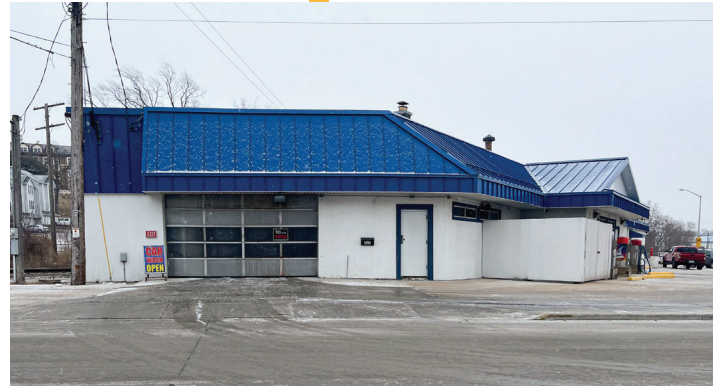
Car wash exit on Main (faces north) Exit is heated to prevent ice build up in winter.
